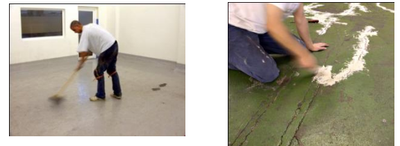
Pic 2. Sweep the floor, remove any highpoints and patch repair or level any cracks or low points.
