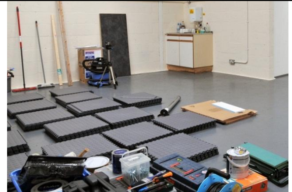
Pic 1. Break down the pallets and allow tiles to acclimatise
