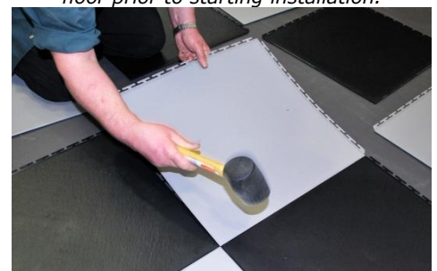
Pic 5. Dont force the tiles, offer up the corner of the tile and gently hammer the joints together.
