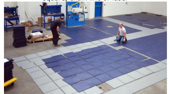
Pic 4. Split the pallet and spread the tiles across the floor prior to starting installation.
